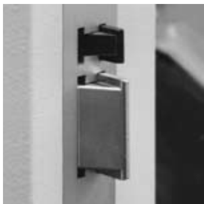
Anti-foutbedieningspal boven dagschoot
